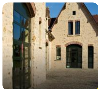
Facade renovation and old buildings
